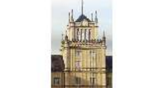
CoE.I, Hauptfassade, Turm, DI009201, BSV-
